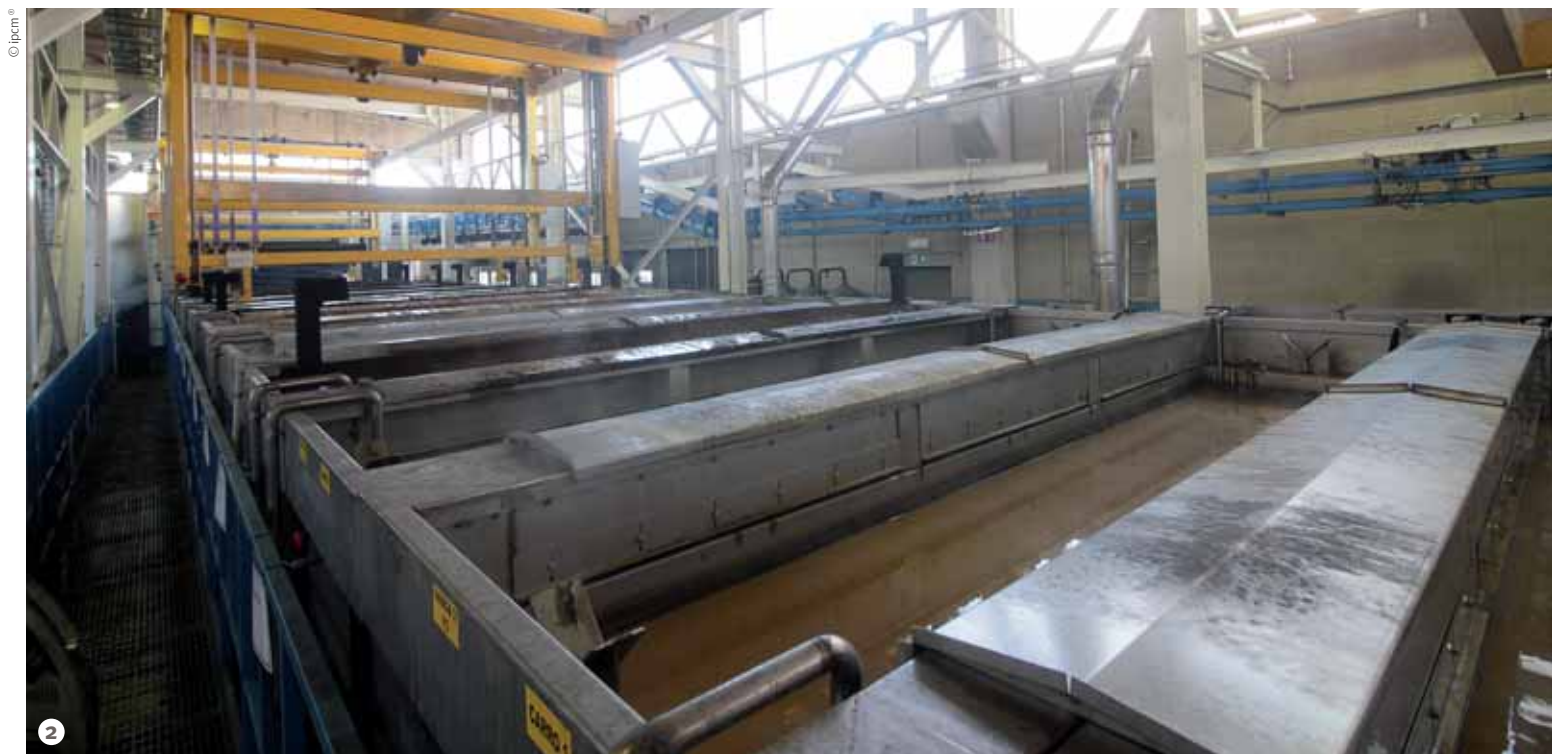
Figure 2: The pre-treatment tanks of the new cataphoresis plant.
