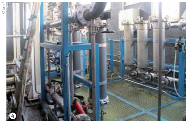
Figure 4: In the foreground, the skid with the 8-inch ultrafiltration membranes installed.
