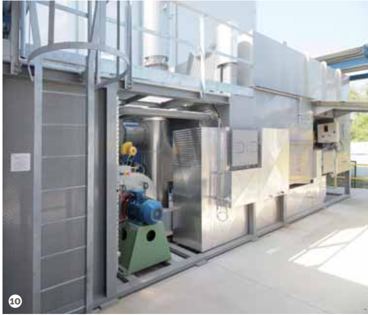
Figure 10: The regenerative thermal oxidiser (RTO) installed by Brofind.
