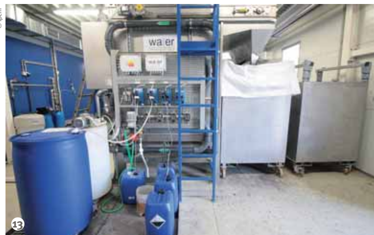
Figure 13: Water Energy's Skimmerflot sludge remover with a flow rate of 15,000 litres/hour.
