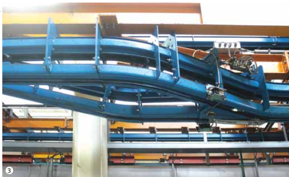
Figure 3: The two-rail conveyor supplied by Futura Convogliatori Aerei Spa has a maximum capacity of 1250 kg.
