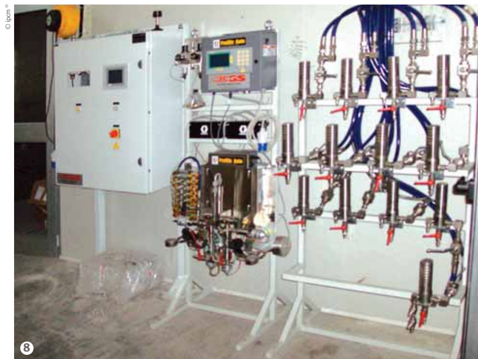
Figure 8: The Promix Auto dosing system previously installed at the Bonfiglioli premises.
