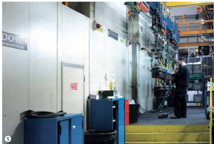
Figure 5: The exterior of the painting system, installed by Tecnofirma (Monza).
