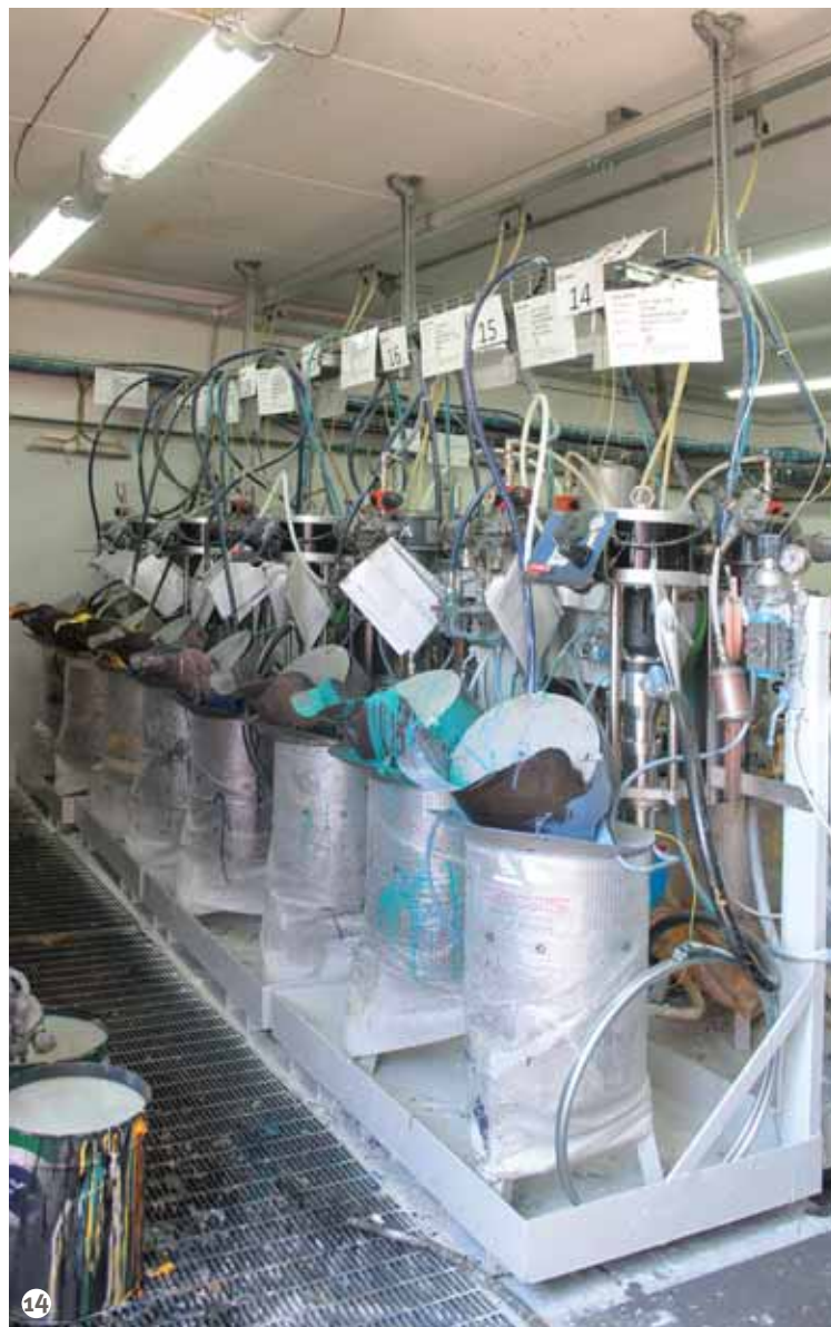
Figure 14: The coating management unit.
