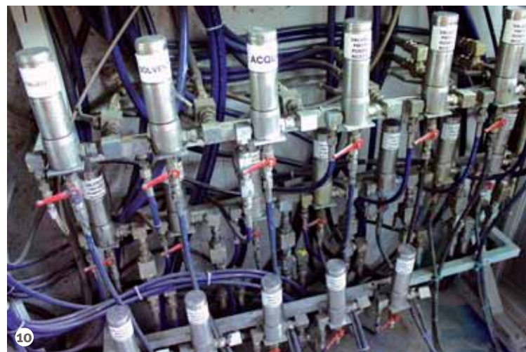
Figure 10: A detail of the pumps.
