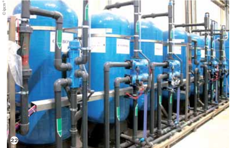
Figure 22: The demineraliser installed by Water Energy.
