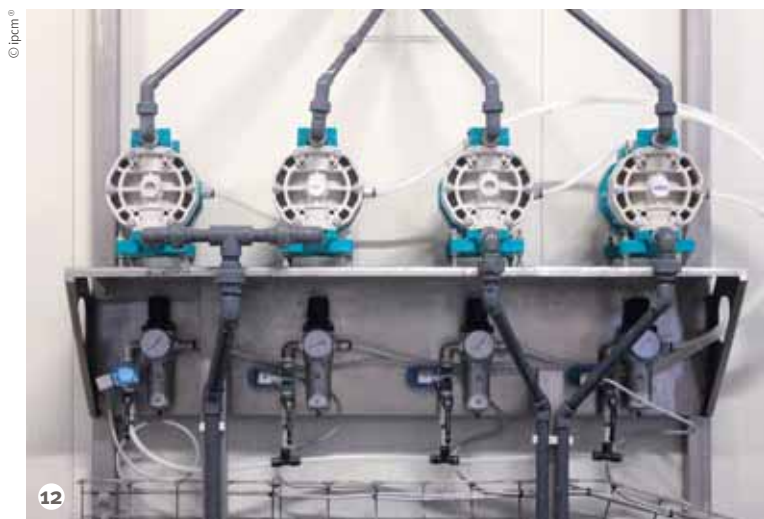
Figure 12: The hydraulic seals' flow panel on the pumps.
