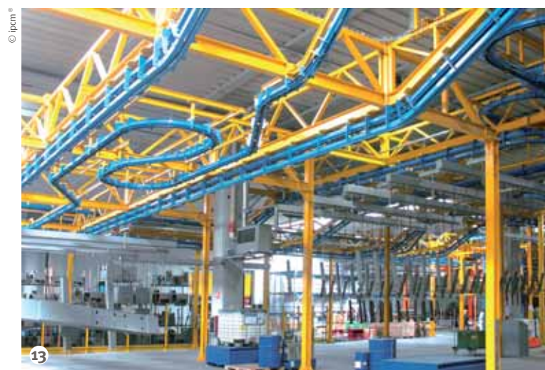
Figure 13: The storage buffer preceding the powder coating application area.
