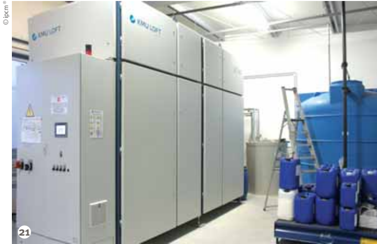
Figure 21: The evaporator provided by KMU Loft.
