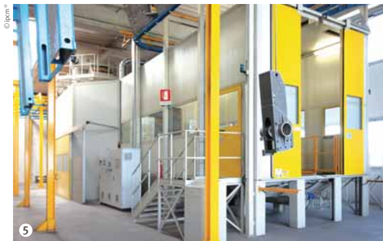
Figure 5: The sandblasting plant.
