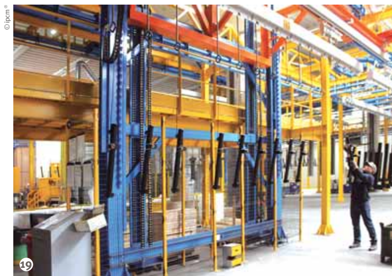
Figure 19: The unloading area.
