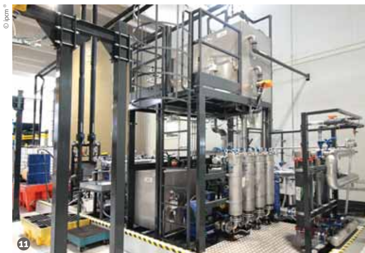
Figure 11: Skids with the anolyte (bottom) and ultrafiltrate (top) tank.
