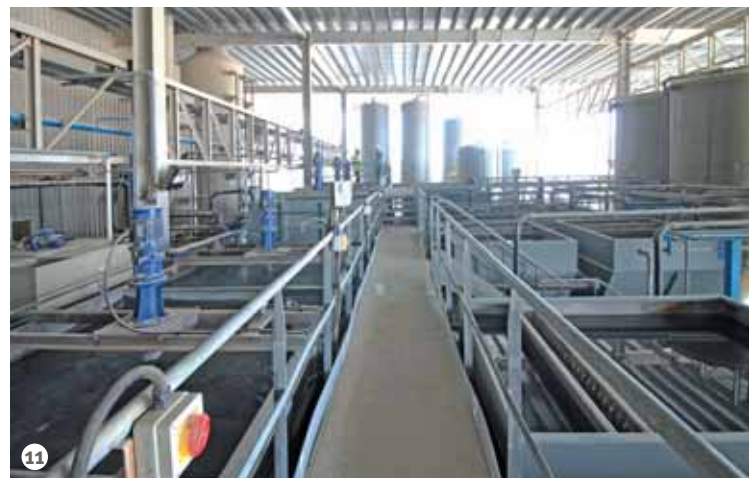
Figure 11: The chemical-physical treatment plant for the coating and anodising processes' waste water.
