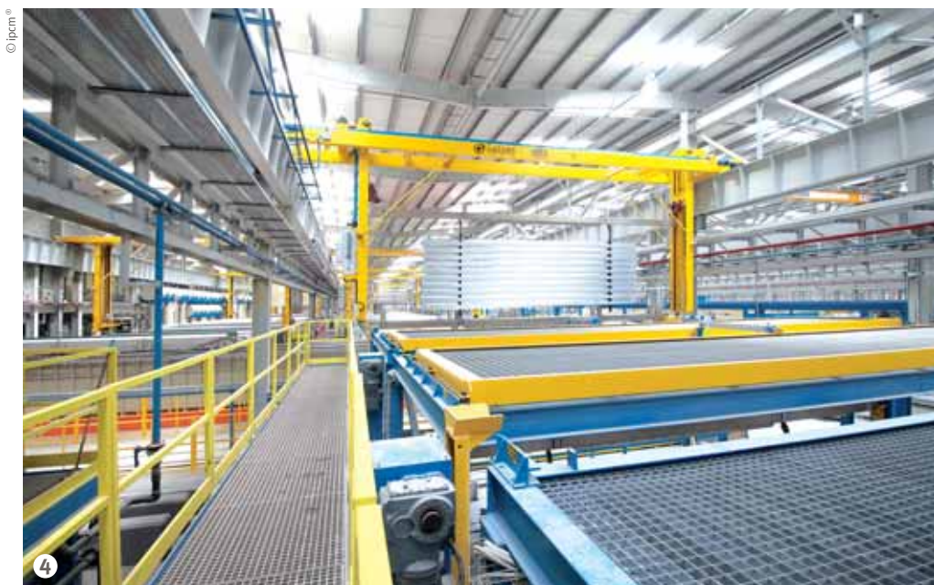
Figure 4: Cisar provided two anodising lines, one for profiles up to 7.2 metres and one for profiles up to 14.2 metres.
