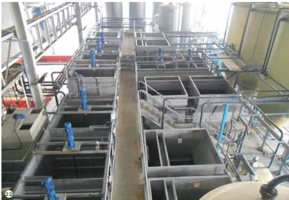
Figure 22: Chemical-physical treatment tanks.
