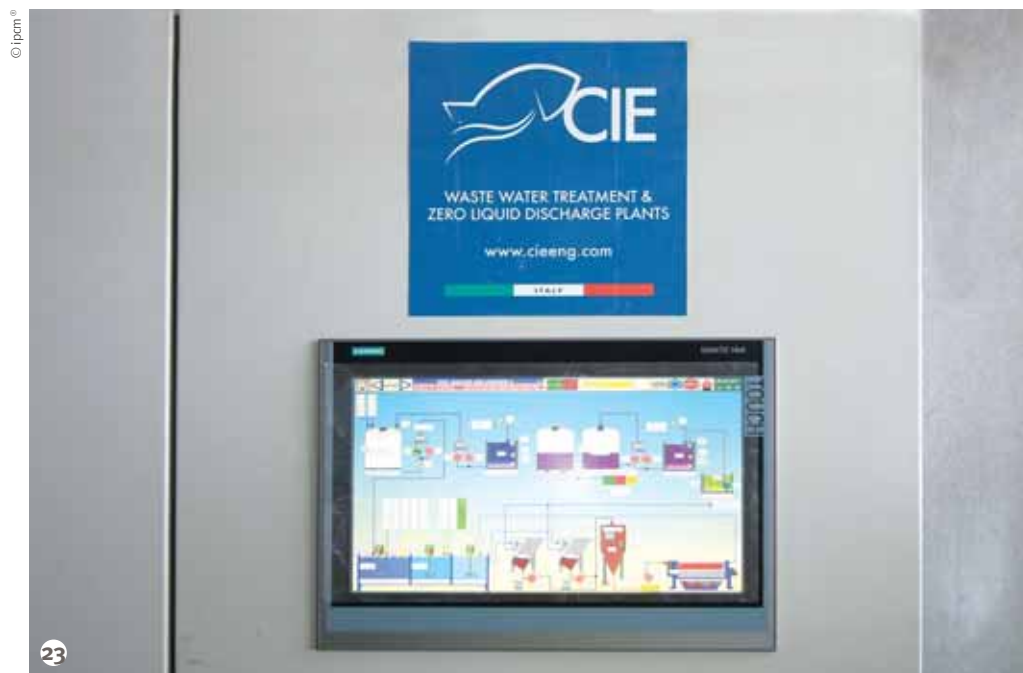
Figure 23: The touch-screen control of the waste water treatment system.
