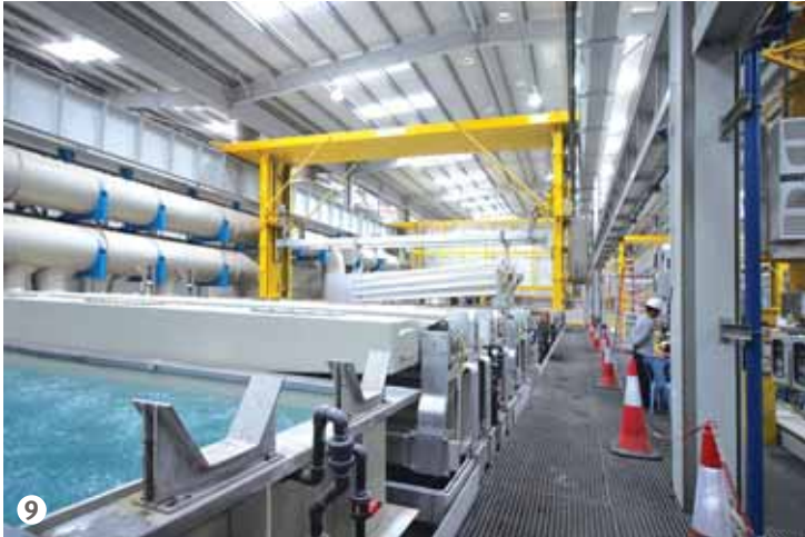
Figure 9: The “short” anodising line.
