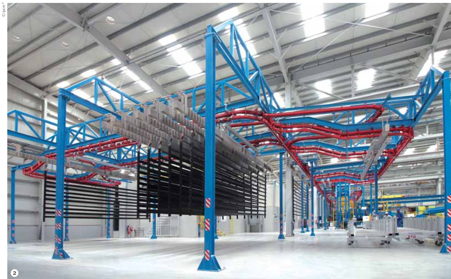
Figure 2: The large size of the horizontal powder coating plant supplied to TALEX by Trasmetal (Milan, Italy).
