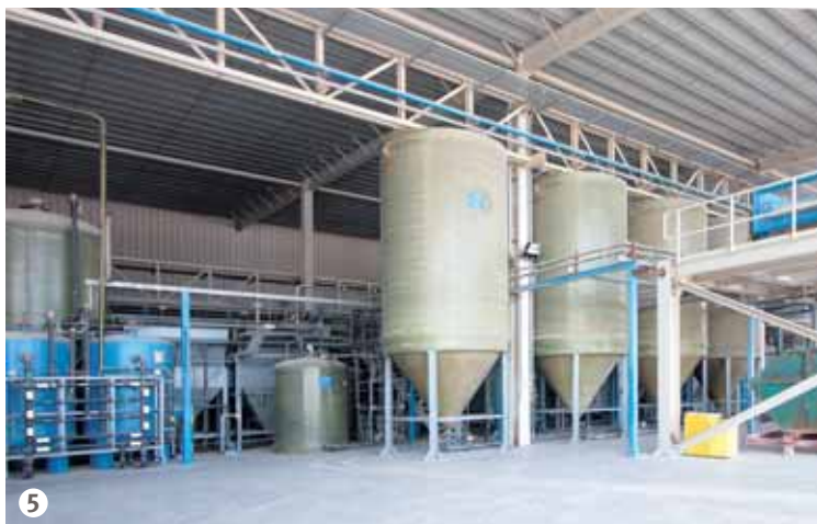
Figure 5: A bird's eye view of the waste water treatment system developed by CIE Srl. In the foreground, the transfer pit area and the buffer area.
