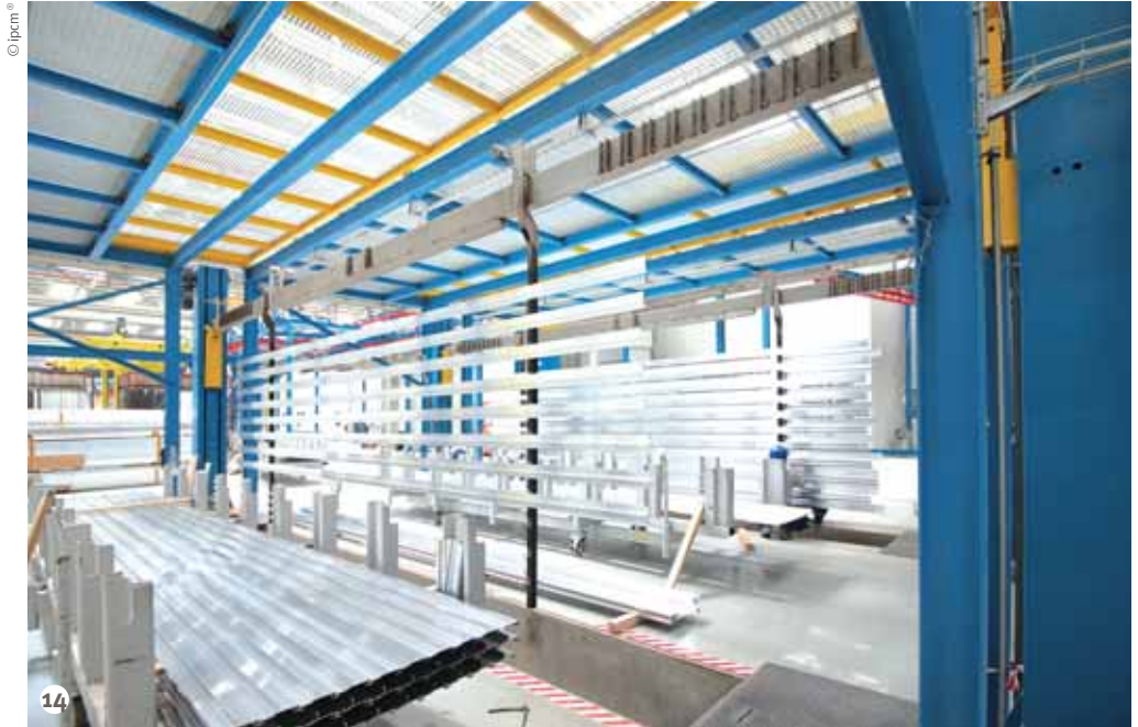
Figure 14: The loading station. The two drop stations can be clearly seen.
